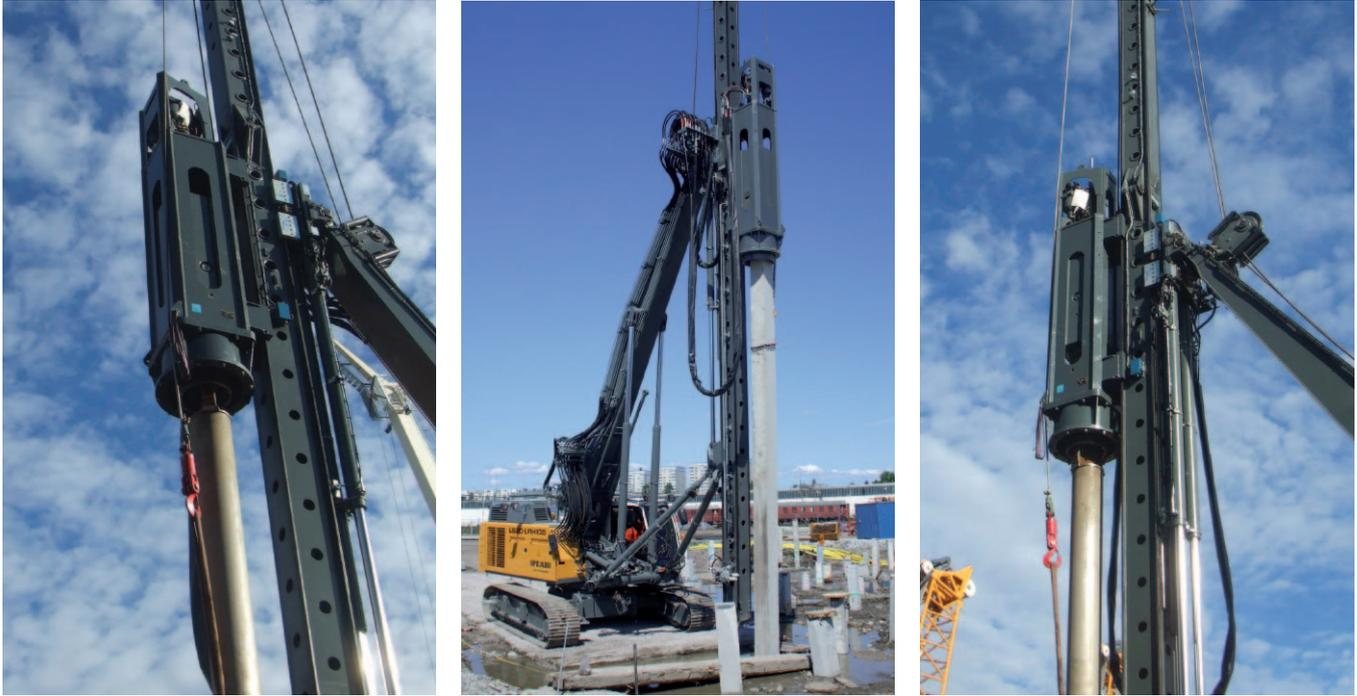
**Above:** The light weight LX hammer gives greater stability to piling rigs, especially in applications where a greater reach is required.
